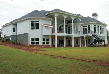
This 9000 sq.ft. Home was built in Conyers, Georgia. Large spans, concrete covered decks and ICF exterior walls set this apart from the rest. Its architecture is Mediterranean. It is magnificent! Steel floor and roof trusses were included as well as interior walls.
