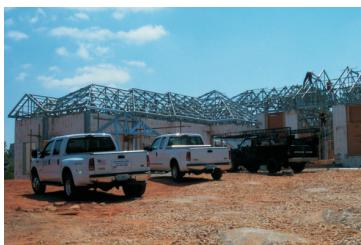
The REPco roof system for ICF has been designed to allow adjustability to set the roof trusses at the proper elevation in spite of the typical irregularities on the top of the ICF concrete wall. Anchor bolts are installed at each truss locations along with a high strength anchor clip. All connections from the anchor to the peak are in shear, which yields maximum strength.
