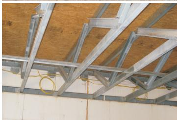
Floor joist and truss systems are fastened to the ICF walls with ledger clips or anchor bolts. Thanks to the high strength rim track, the anchor clips can be located between the trusses or joists eliminating interference at the truss locations. Floor trusses are top bearing, making layout and installation a snap.
