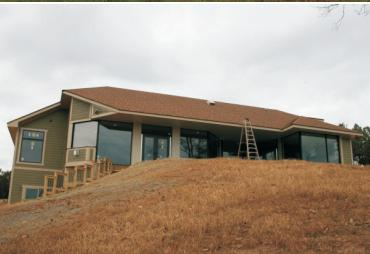
This 6,000+ sq.ft. Contemporary home was built in Ballground, Georgia. It features a large cantilevered roof over floor to ceiling mitered glass window walls. Minimal bearing points necessitated large girder trusses and tube steel columns. All engineering by REPco.
