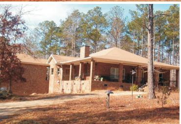
This home has 4500 sq. ft. plus a basement, complete with an in-law suite. It incorporates steel frame floor and roof trusses as well as interior walls. An open floor plan is accented by a large Great Room. The roof trusses are 40'+ clear span.
